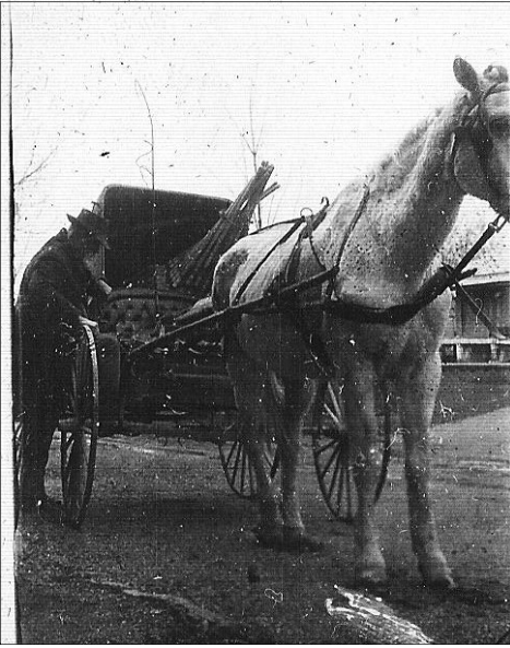
Photograph of Sam Crabb loading his horse drawn wagon with Shively's Brooms. The Millmont Railroad Station is in the background.
